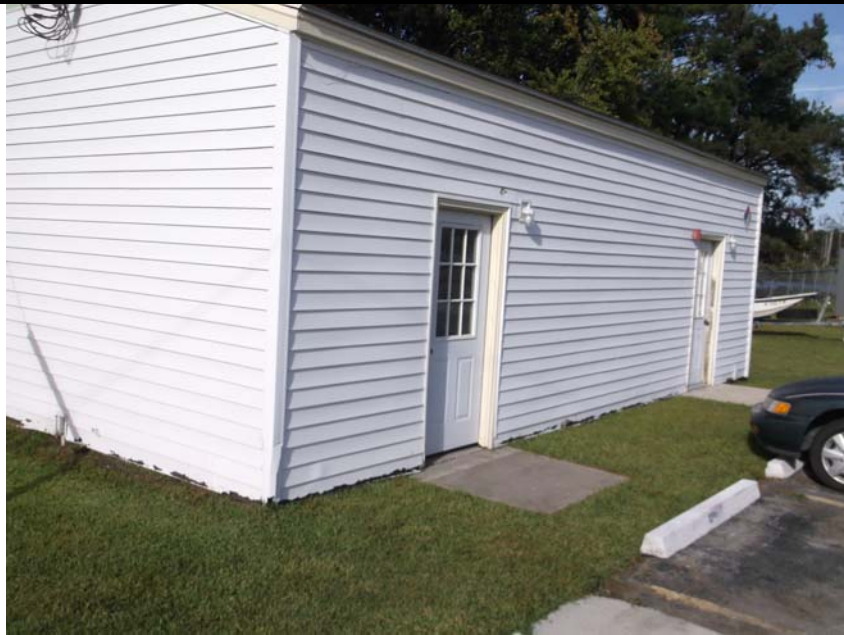
Photo 1: Exterior view of the Bos'n Hole building (OS2).
